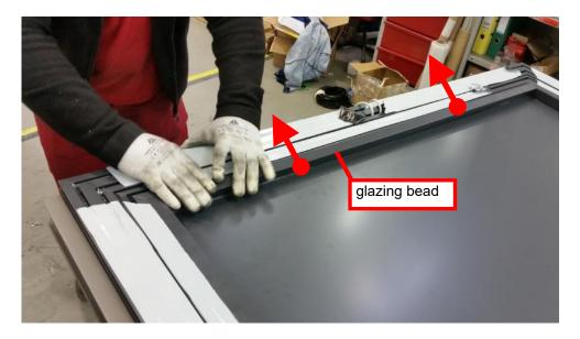
4. Install gaskets between glazing beads and the glazing.
